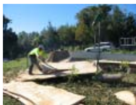
Above: Camphor on site is felled and sawn into slabs on Lot 4, to be used once it's seasoned.
